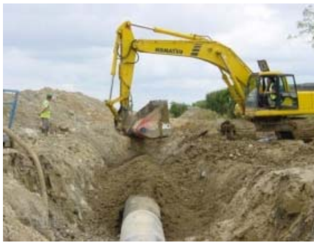
Picture 4. ALLU SM filling pipeline in Ireland
